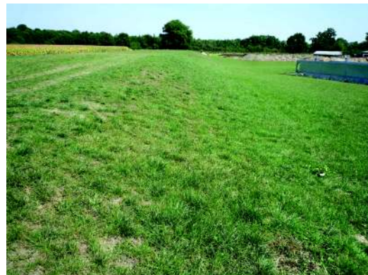
Figure 5.30: Photo de la pente
